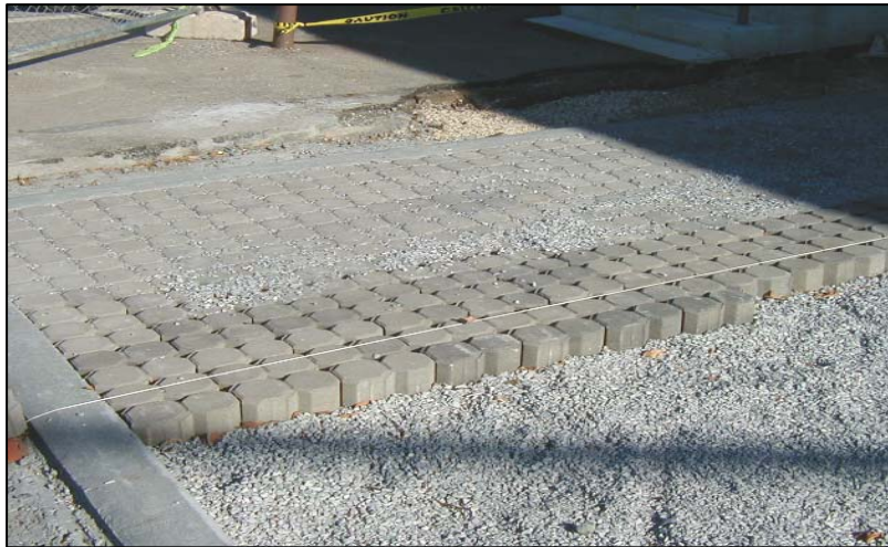
Figure 1: Installation of a Permeable Paving System
