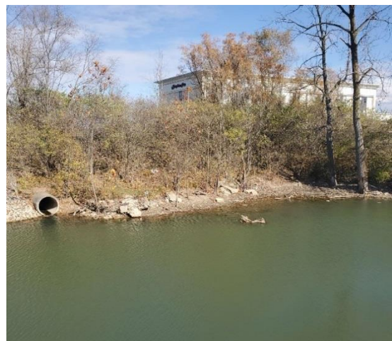
42-inch outfall at north bank of pond
