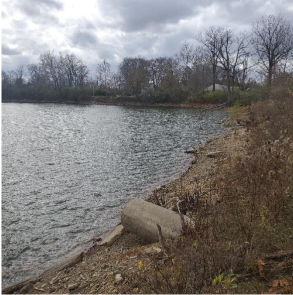
24-inch pipe at north side of Burnside Pond
